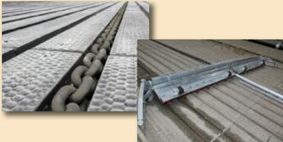
Ammonia emission reduction flooring systems
