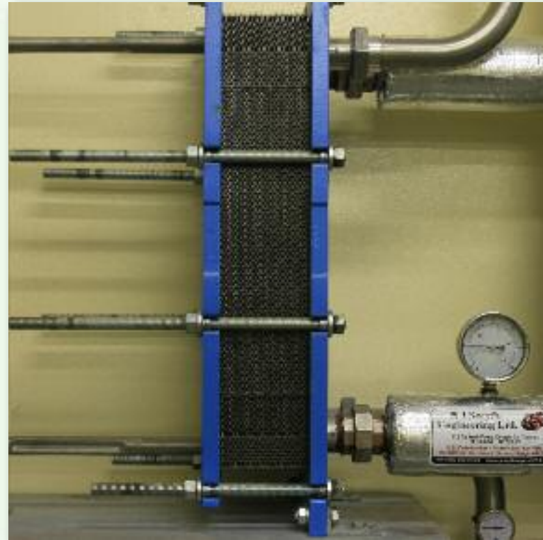
Plate heat exchanger used to cool the milk.
